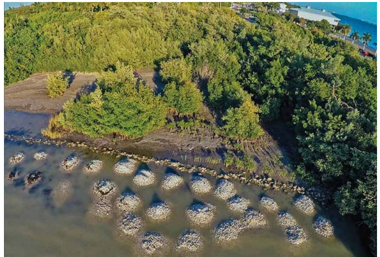
Living shorelines in Punta Rassa, FL. Photo © www.floridalivingshorelines.com
